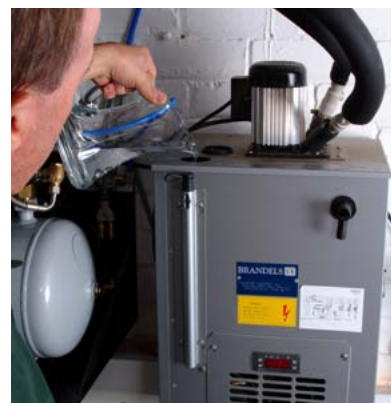
Top up the cooling unit every six months to keep the beer in the lines at cellar temperature.
